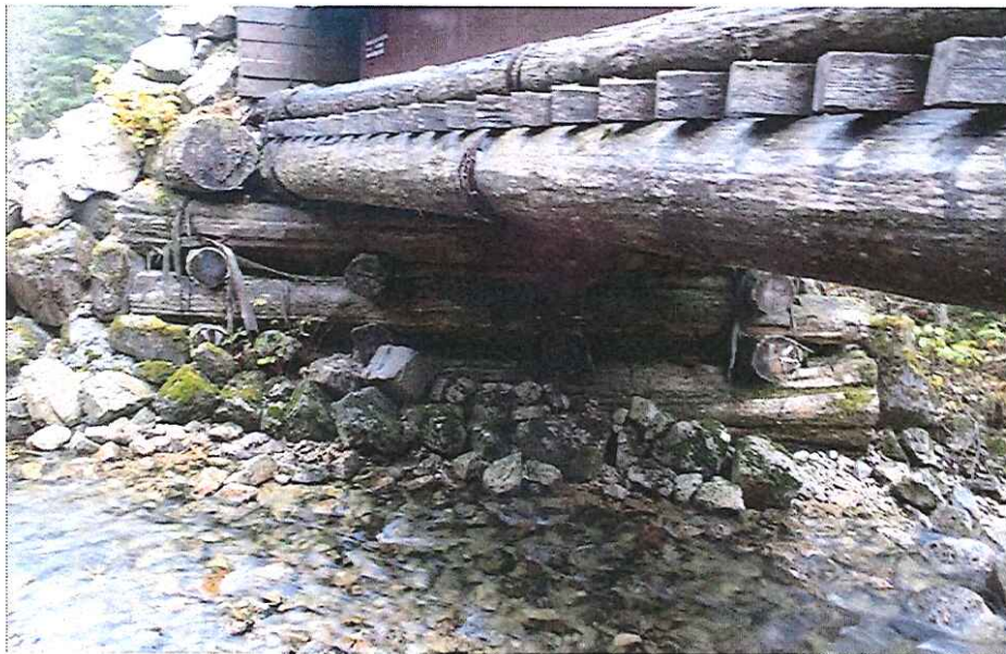
CK2270 Left Abutment
