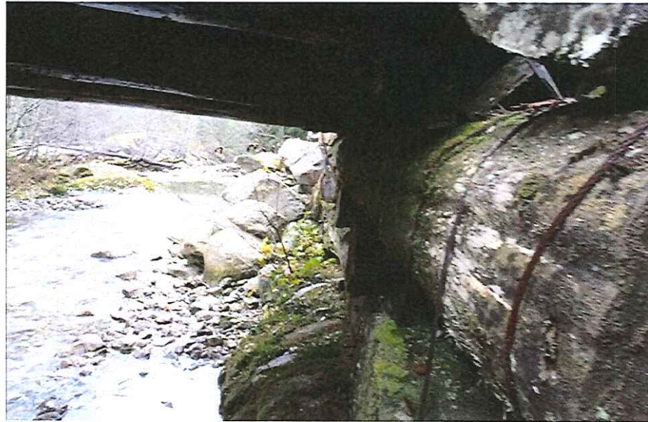
CK2270 Right Abutment Crip
