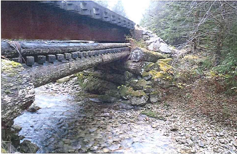
CK2270 Right Abutment
